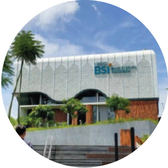
Masjid BSI Cipali
